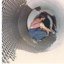
Laying of refractory lining
